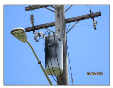
Photograph 18. One pole-mounted transformer was observed to the south of the subject property, along Atbut Lane and at an apartment building. Black staining was visible on the exterior of the transformer (09 May 2019).
