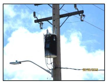
Photograph 17. One pole-mounted transformer was observed to the northeast of the subject property, along University Avenue. Black staining was visible on the exterior of the transformer (09 May 2019).
