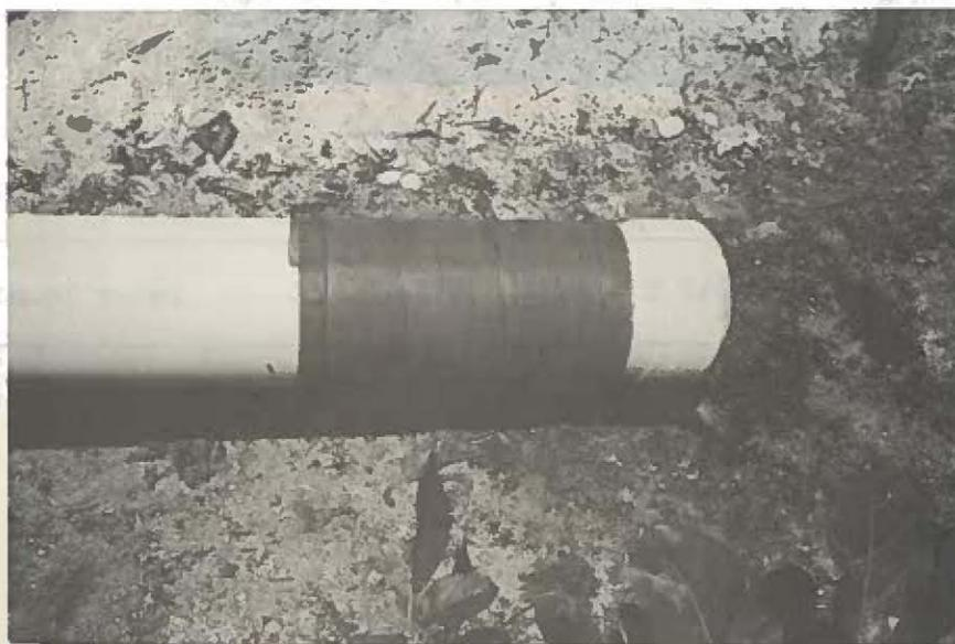
Figure 7. Pipe cap and fiberglass window screen in place on bottom end of well casing.
