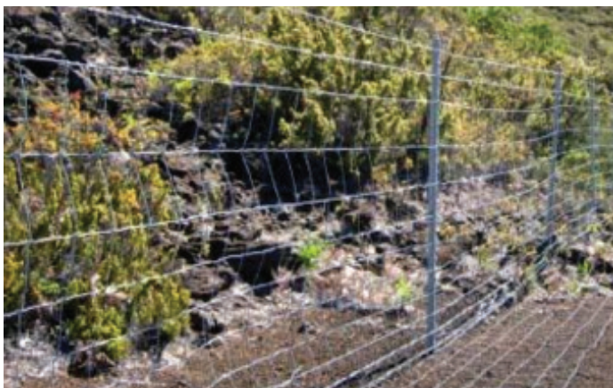
Figure 1 A ground skirt (the portion of the fence laying flat on ground) on the outside of an exclusion fence keeps feral pigs and dogs from digging underneath it. Source: Mauui Now
