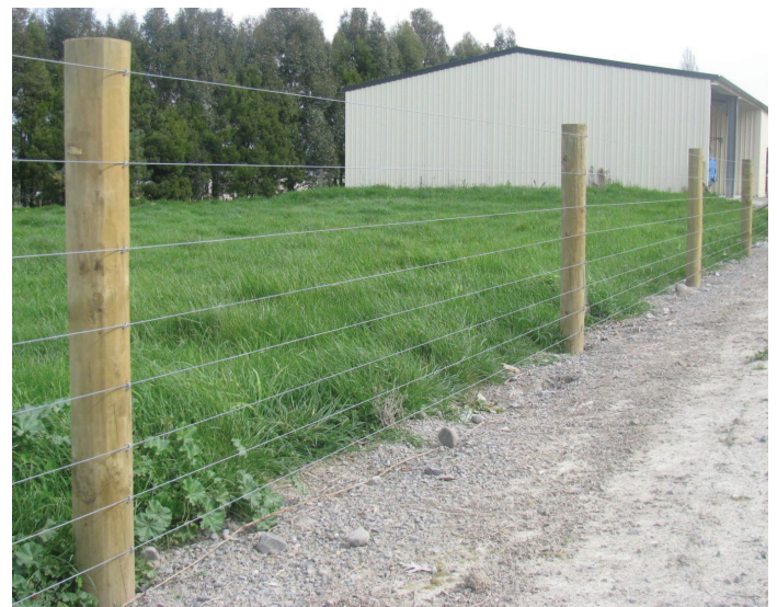
Figure 2 A multi-strand wire fence with wooden posts. Source: Conventional Farm Fencing , n.d.
