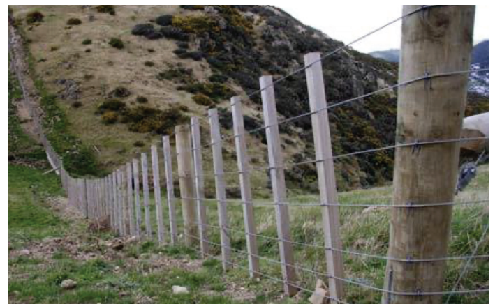
Figure 3 A multi-strand smooth-wire fence with battens installed between fence posts. Source: Conventional Farm Fencing , n.d.
