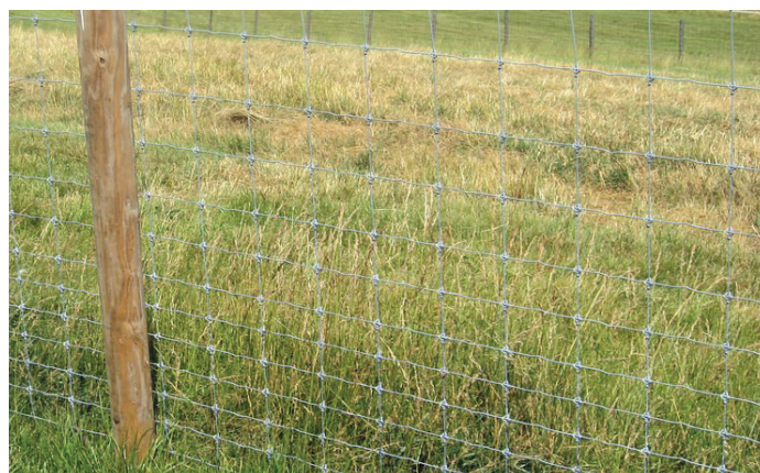
Figure 6 Woven wire fence. Source: Cornerstone Fencing Ohio ( cornerstonefencingohio.com )
